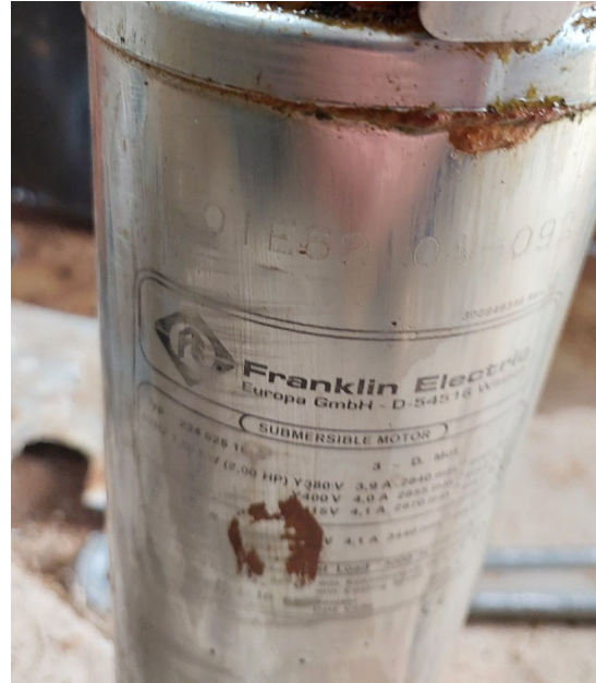
Identification plates as noted on submersible motor and wet end.
