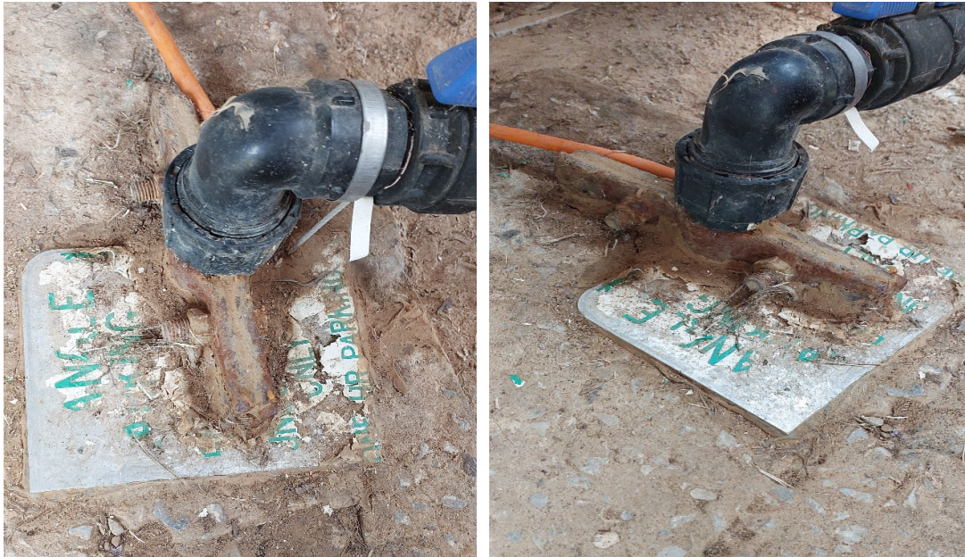
Unsealed headworks as viewed from surface.
